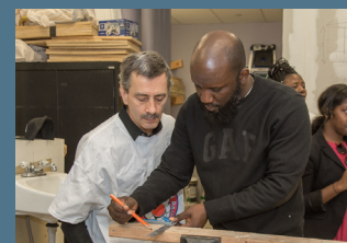
Residents Enrique Arrazola (left) and Elliott Byran (right) prepare to solder a copper supply line at the Resident Training Academy.
