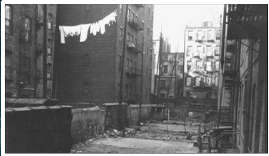
Before A view of the backyard at First Houses prior to the construction.
