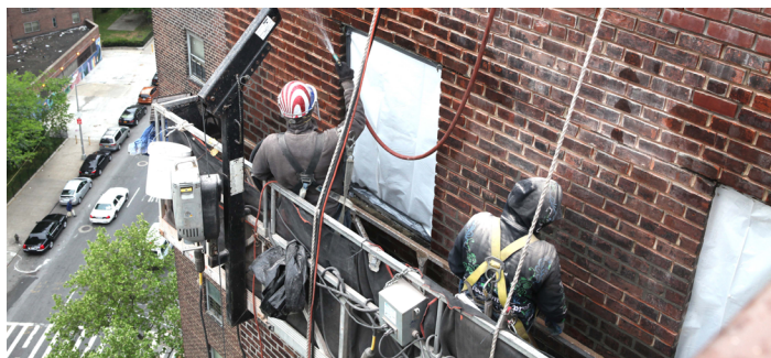
Exterior masonry work at Lincoln Houses included brick restoration, re-pointing, and waterproofing on the facade, and other work to seal the building envelope.
